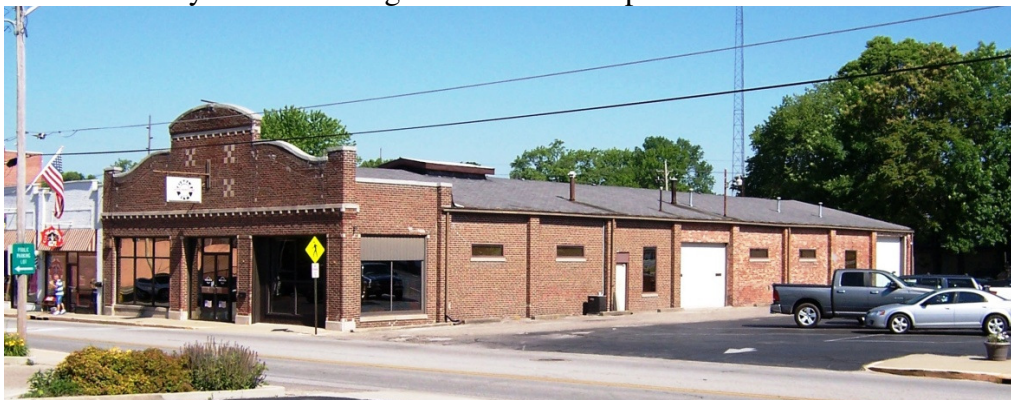
The building at 172 W. Main Street in Greenwood was once a Dodge/Plymouth dealership.
